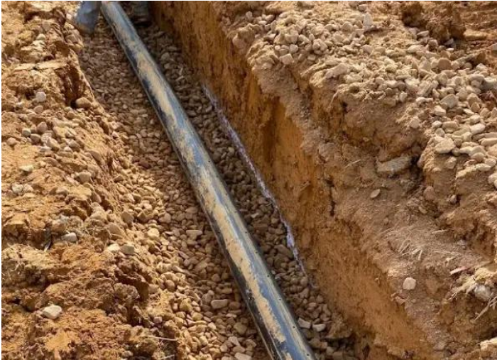
Perforated pipe being buried in gravel filled trench that will extract gas along the sidewall. Courtesy of City of Bristol
