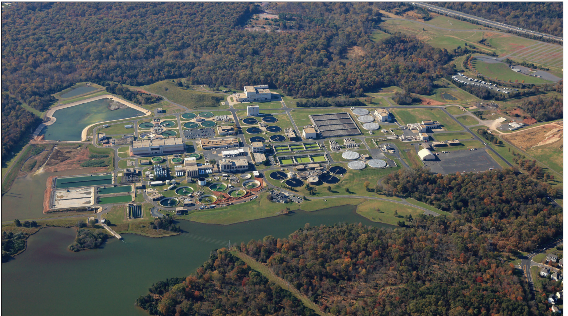
Manassas and Prince William County are planning to expand their wastewater capacity at the Upper Occoquan Service Authority.
