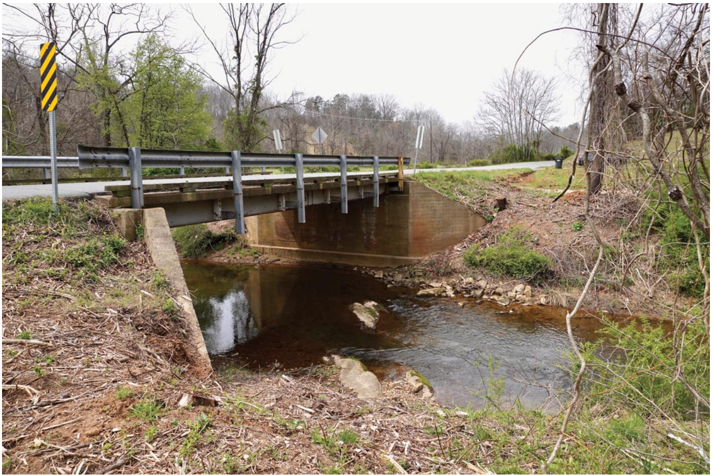
VDOT plans to upgrade this bridge on Plank Road over the Mechums River, just west of Batesville. Photo: Lisa Martin.
