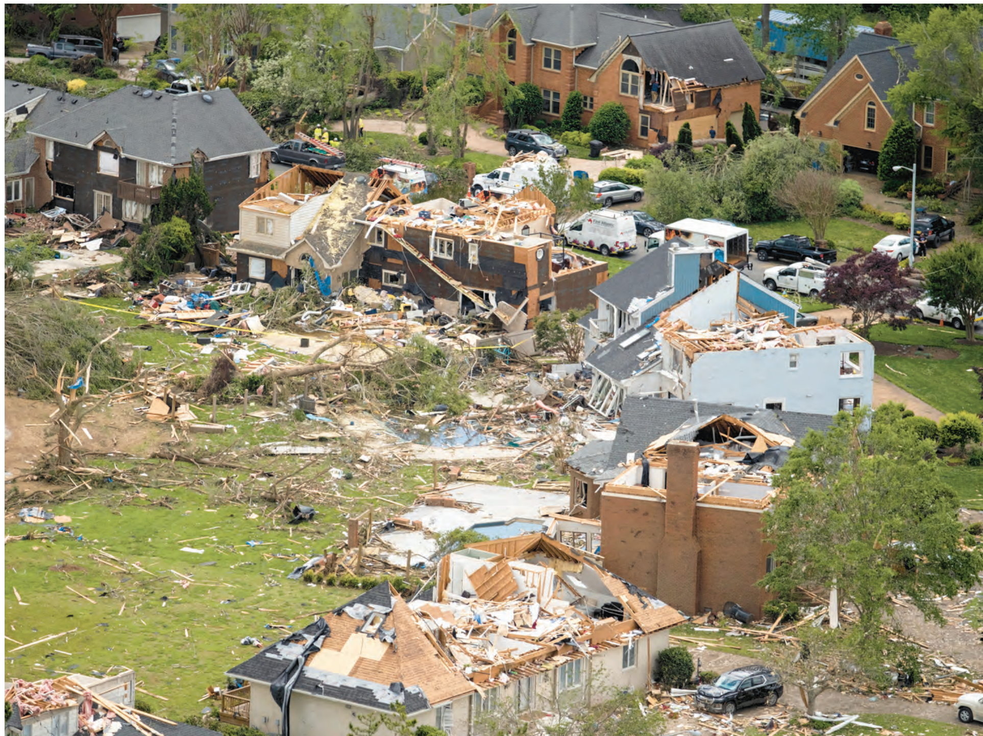
A late-afternoon storm Sunday brought severe damage to the Great Neck section of Virginia Beach. BILLY SCHUERMAN/STAFF
