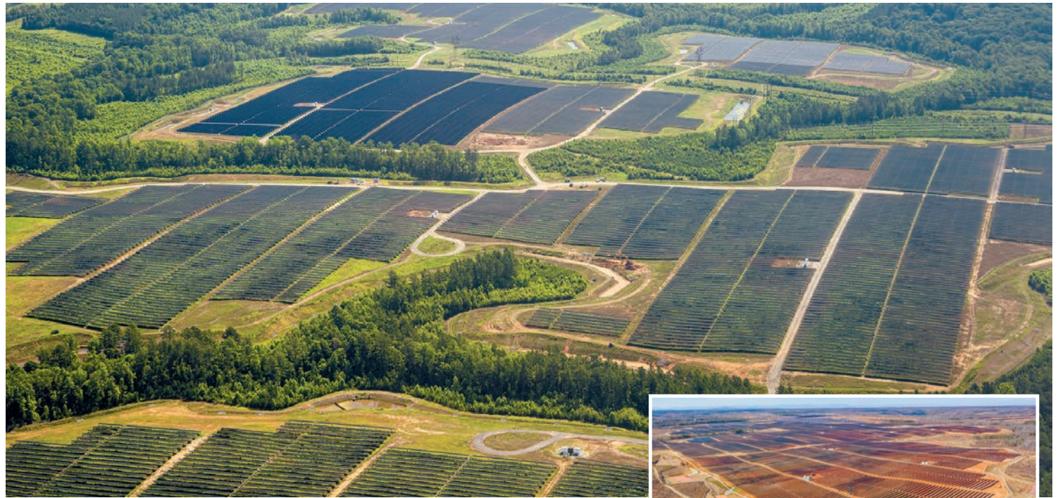
Above: This solar facility, built by Utah-based Sustainable Power Group, or sPower, in Spotsylvania County, VA, covers more than 6,000 acres.
