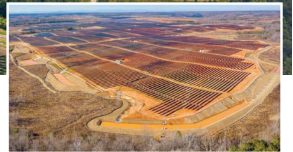
Right: Exposed soil was pervasive at the site in early 2021, before vegetation was planted to reduce runoff. (Photos by Hugh Kenny/Piedmont Environmental Council)
