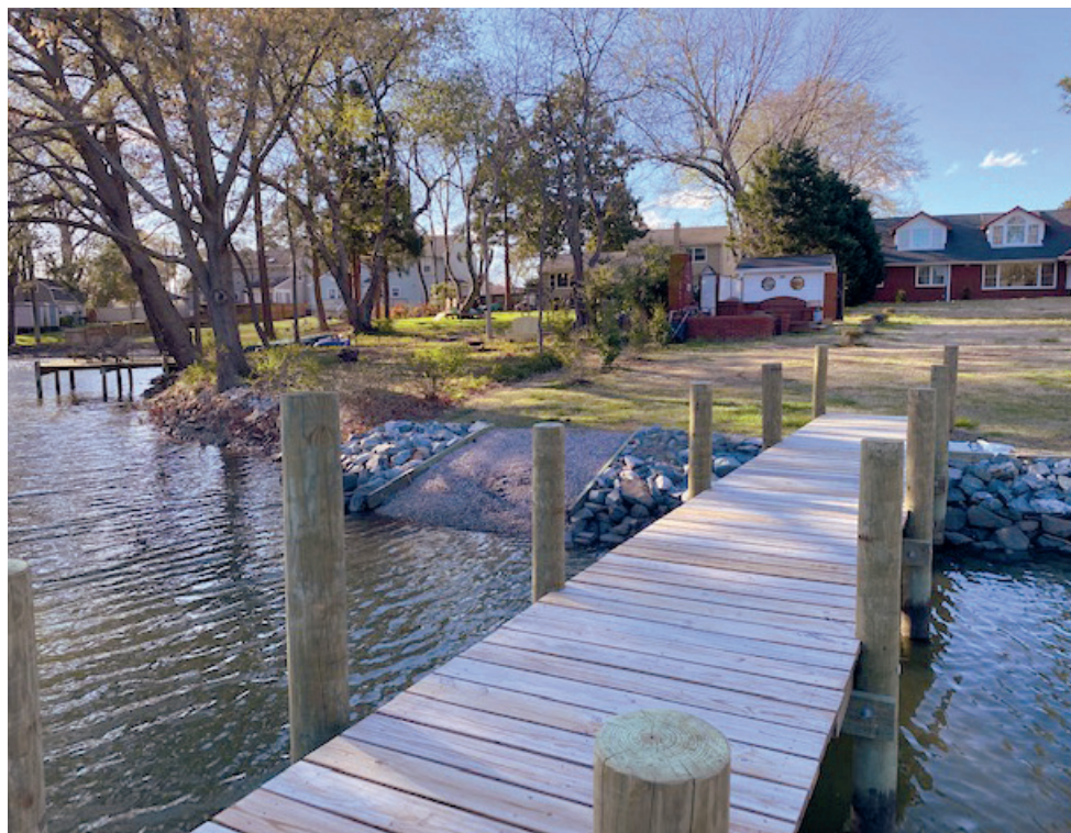
A contractor who built a permitted pier along this shoreline in Hampton Roads, VA, added stone and a gravel kayak ramp without getting a necessary permit required under the state's living shorelines law. The landowners tried to correct the issue by adding living shoreline elements but were denied a permit three times. (Courtesy of Mary Swift)
