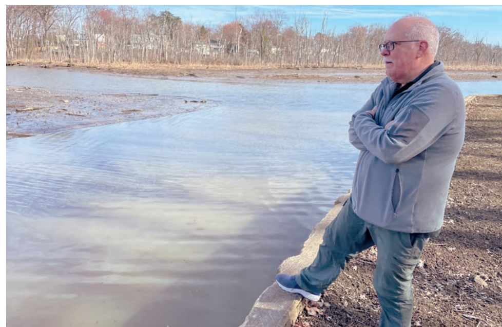
Brian Jones' efforts to repair or replace the seawall along his property in Alexandria, VA, met with complications under the state's new living shorelines law. (Whitney Pipkin)
