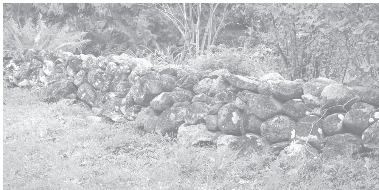
This old dry stacked stone wall is more of a jumble of stones without too much thought as to the placement of the stones.
