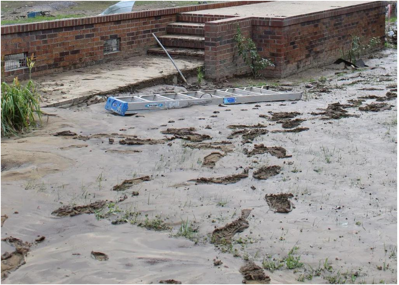
Flood damage in the Pilgrim's Knob section of Buchanan County. Photo by Lakin Keene.
