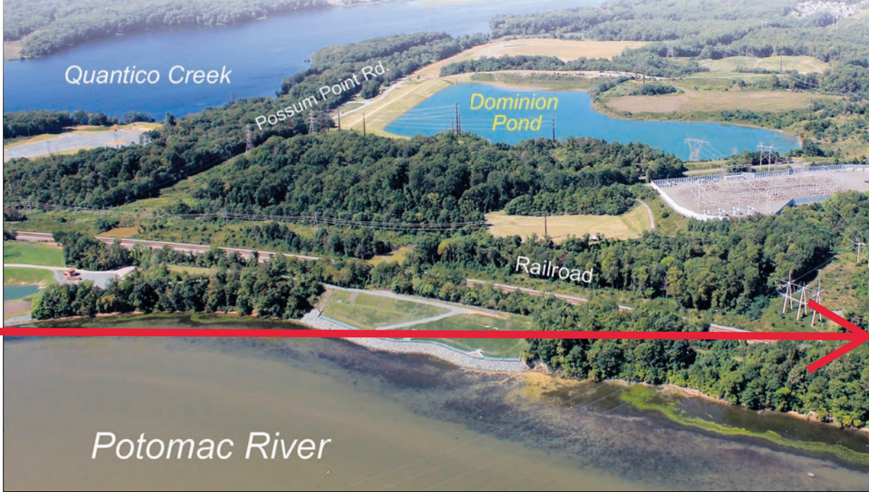
The current coal ash pond at Dominion Energy’s Possum Point Power Plant site is seen in this aerial photo taken in September. Dominion’s proposed landfill would be just west of the pond site. The power plant itself is along the Potomac River, just outside the photographed area. (See additional photos, Page 6).
