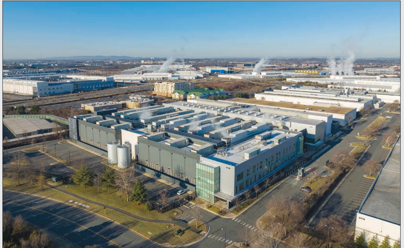
This photo, taken from a drone in February, shows a few of the 25 million square feet of data centers that have been built in the Ashburn area of Loudoun County. VANTAGE POINT DRONE | FOR INSIDENOVA
