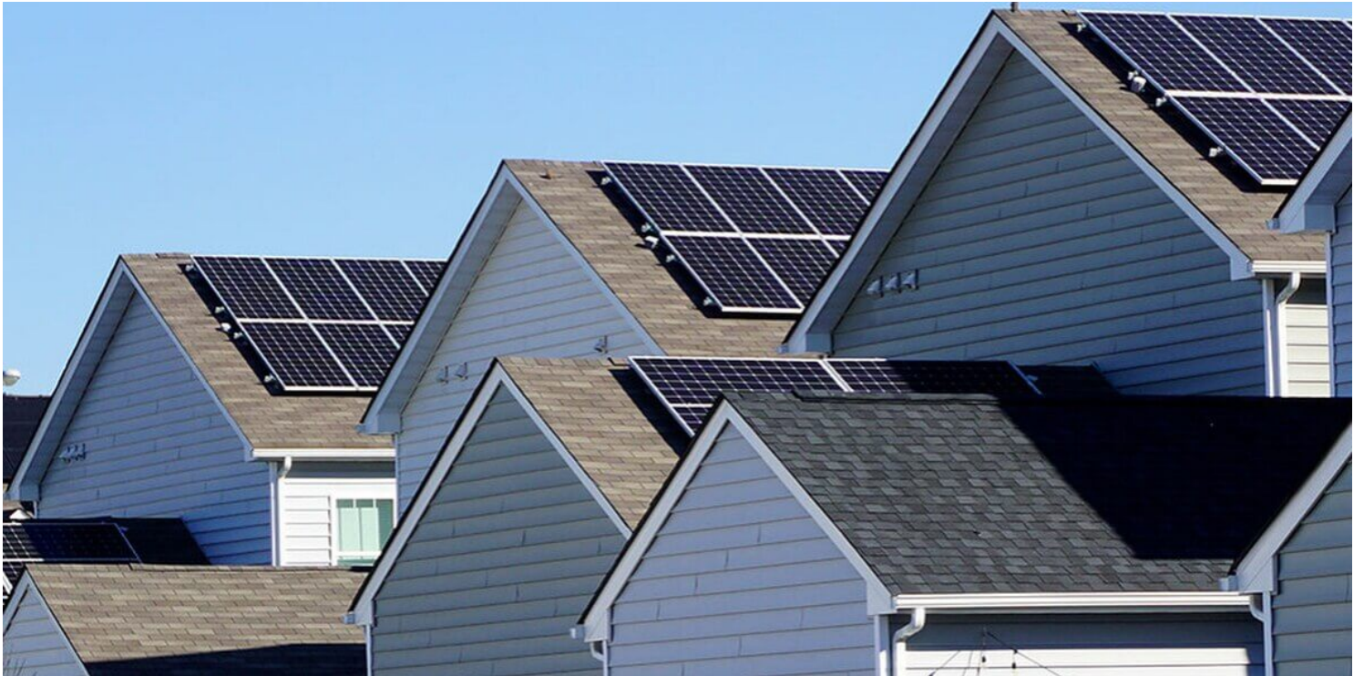
Rooftop solar panels. (VCU Capital News Service)
