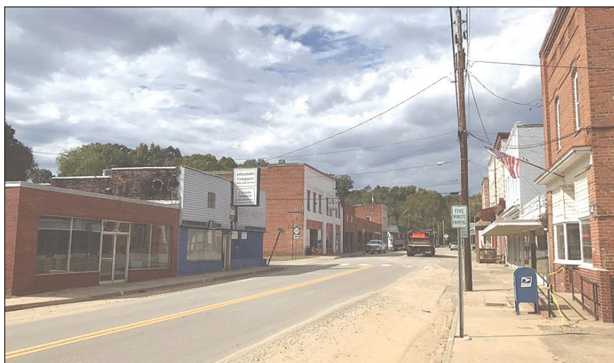
The Town of Drakes Branch has been awarded close to $1 million to help with demolishing buildings that were damaged in 2018 during Tropical Storm Michael.
