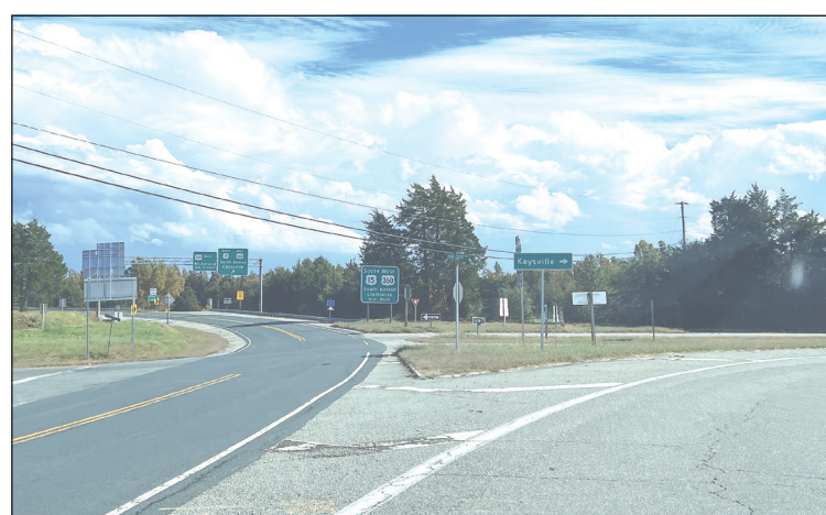
Starting next year, drivers will begin to encounter construction at the intersection of Routes 15 and U.S. 360 as VDOT moves forward with a roundabout for the area.
