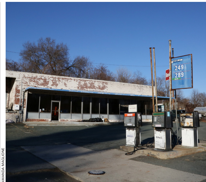
Charlottesville Oil sits on a 1.31-acre parcel on Ivy Road. Albemarle County assesses the land at $922,700, and the three structures there at $199,100. An adjacent 1.21 parcel, where empty semi-trailers are often parked, is assessed at $869,700.
