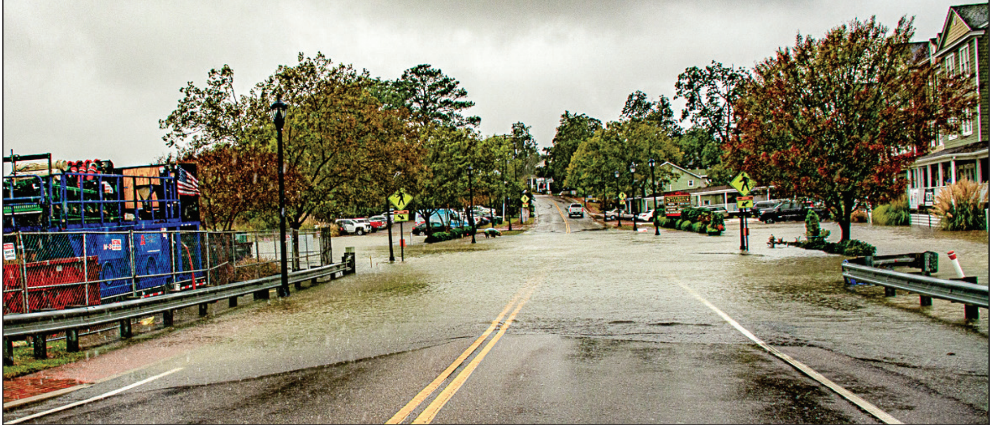
South Church Street at the Cypress Creek Bridge was closed to vehicular traffic during Saturday’s high tide. (Photo courtesy of Joe Lupton)
