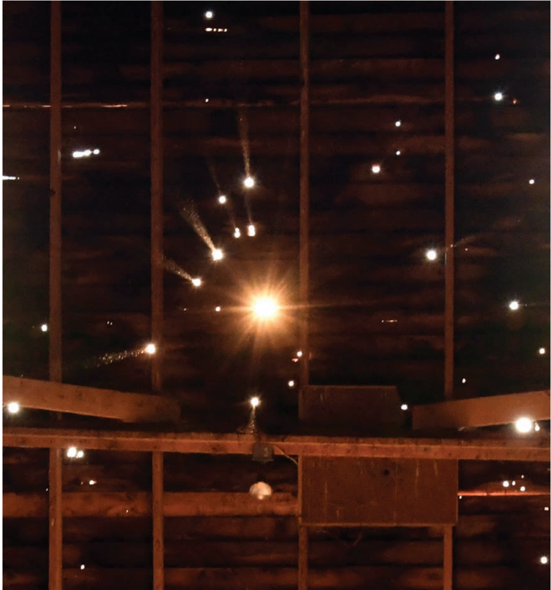
Sunlight pierces through holes drilled by carpenter bees and project large round dots on the barn’s opposite wall.
