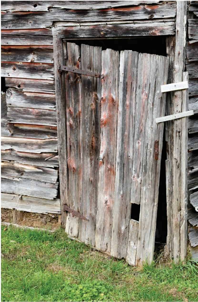
Time has taken away the red paint and added a weathered gray patina. Openings were cut in barn doors to allow cats inside to control rodents.
