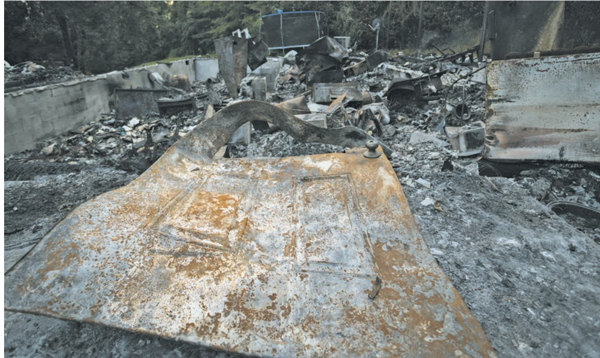
The former door to the home's main entrance.
