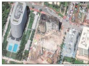
In this satellite image provided by Maxar Technologies heavy-lift cranes are used to aid in the search and recovery operation at the partially collapsed Champlain Towers South condo building on Saturday in Surfside, Florida.
