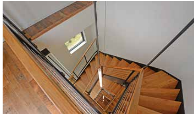
The staircase that spirals the length of the four-story town house in Manchester is at the heart of the architecture. There's also an elevator for added convenience.
