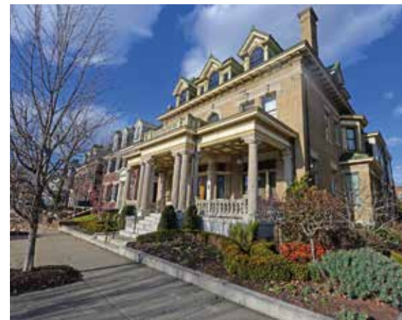
The 10,000-square-foot house at 2710 Monument Ave. was vacant for years until renovated by Paul and Julie Weissend. It had been the Senior Center of Richmond.
