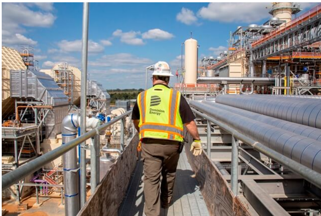
A Dominion Energy employee surveys the natural gas-fired Greenville County Power Station which began commercial operations in December 2018. (Dominion Energy news release)
