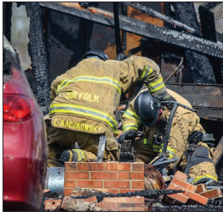
Suffolk Fire and Rescue crews battled a residential structure fire Monday morning on Five Mile Road.
