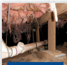
Crawl Space Repair
